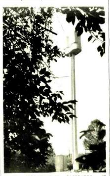
THESE MODERNISTIC CANISTERS will house seven bi-directional transmitter and receiver systems, plus a standby, together with antennas and interconnecting equip-
